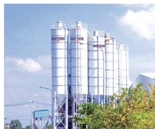
Trạm trộn bê tông / Mixer Plant Quatity: 09 units Capacity: 30 - 120 m 3
