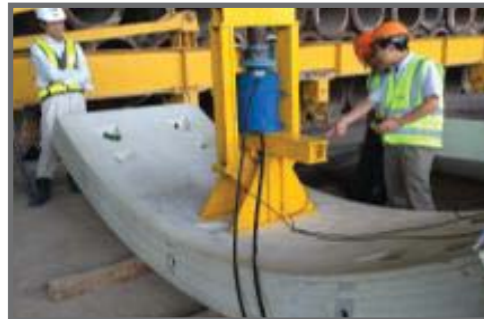
KÉO LỖ CẦU (LỖ BƠM VỮA) Lifting Hole Stressing (Hole For Mortar Pump)
